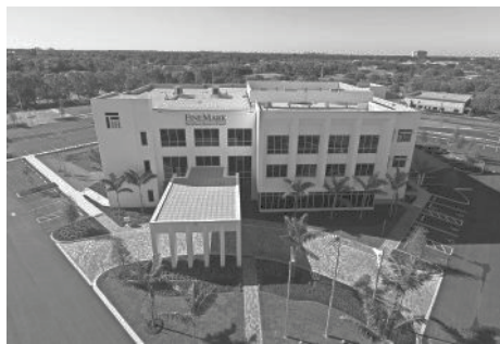
FineMark National Bank & Trust’s new headquarters at 12681 Creekside Lane is in Riverwalk at Whiskey Creek corporate park in Fort Myers.
